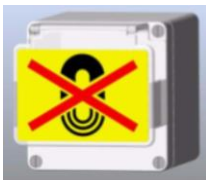
Prisma scan room quench button is behind the plexiglass cover
